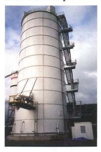
At the end of 2002 Van Aalst Bulk Handling BV delivered and installed a 5000 ton storage silo for cement. The silo has a diameter of 13 meters and a height of 32 meters.
